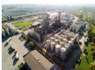
Temix Oleo manufacturing plant in Calderara di Reno (Italy)
